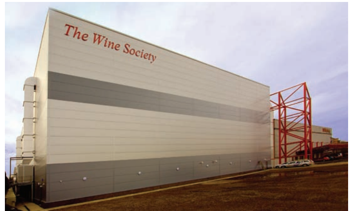
Wine Society Climate Controlled Warehouse, Stevenage, Hertfordshire Architect: Vincent and Gorbng
